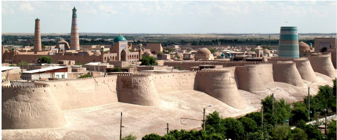
Figure 2. The wall of Ichan Kala
