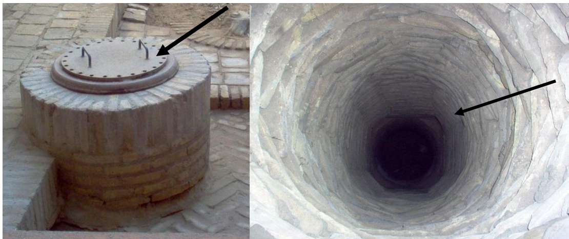
Figure 7. The top part of the well was rebuilt with burnt bricks in the independent years, and the inner part was remained as it was before
