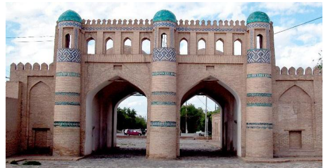
Figure 3b. General view of the Kosh-Darwaza gate
